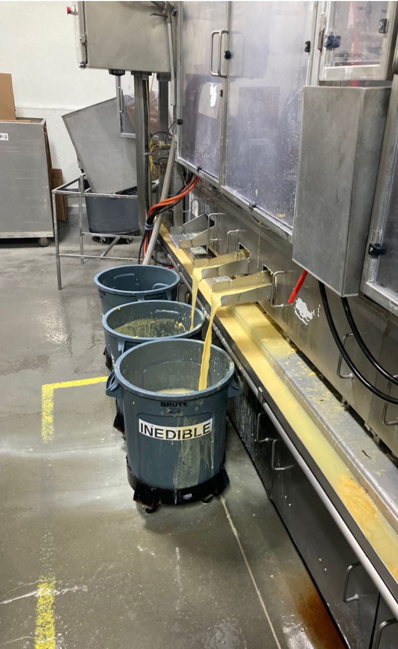
Kozy Shack Facility in Turlock, CA.
